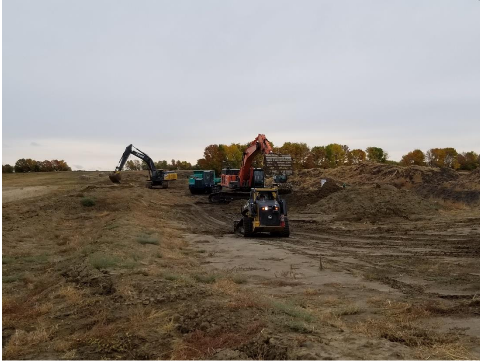
Final Clean-up crew backfilling mud pits from the past Vac trucks dumping the mud.
