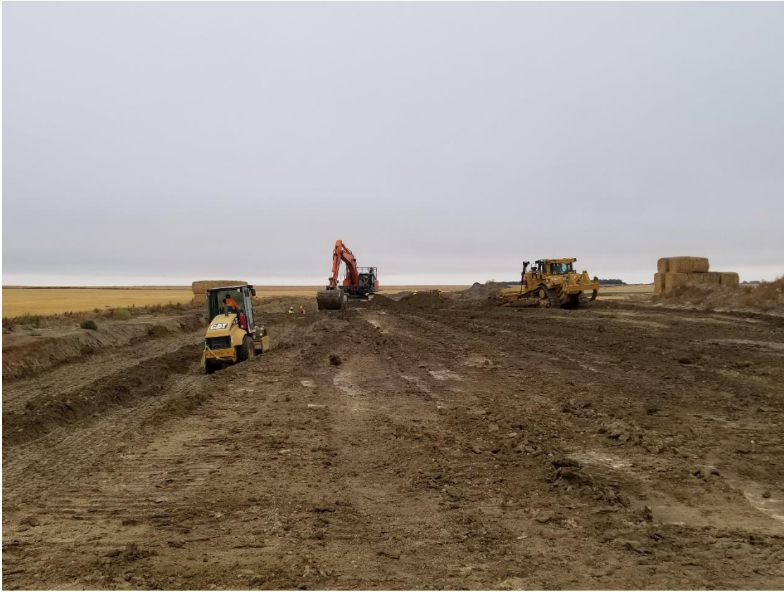
Final Clean Up crew backfilling an old testing point.
