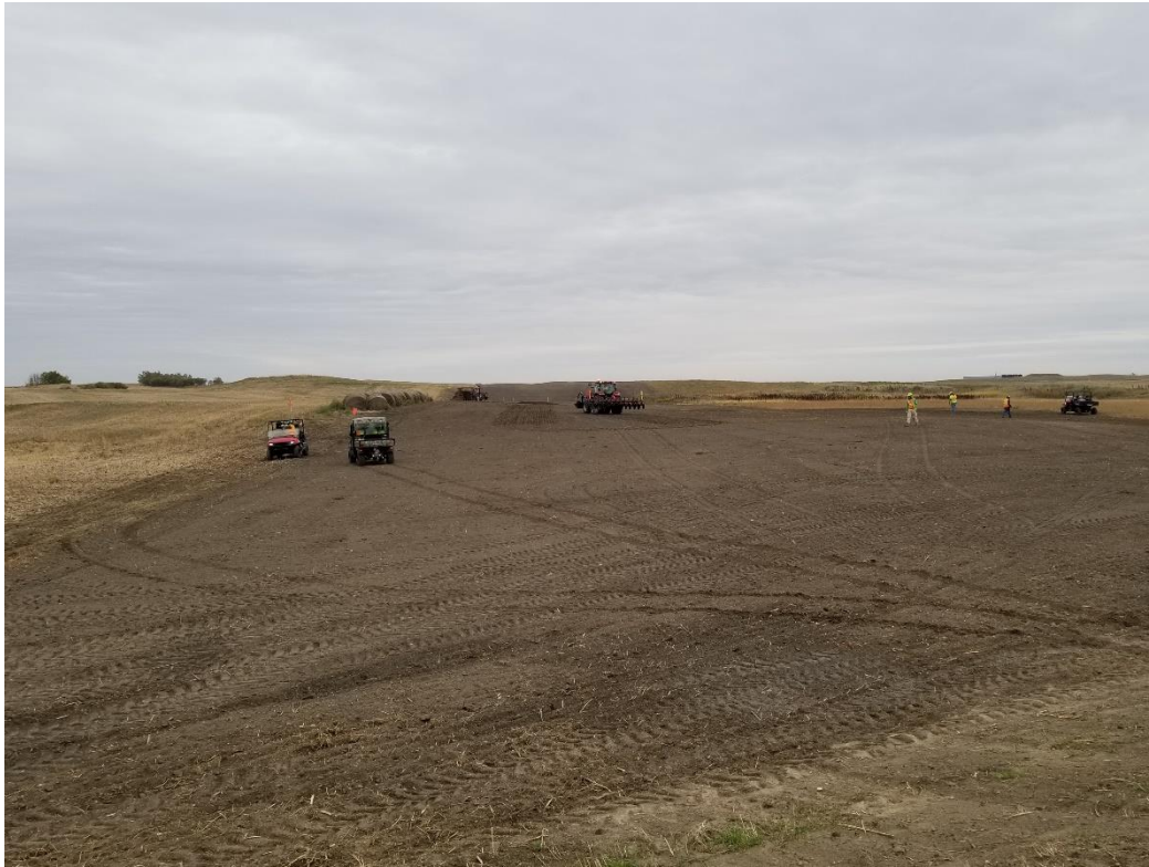
Straw crimping crew preparing to spread the straw, and making sure the ground is not too wet and muddy.
