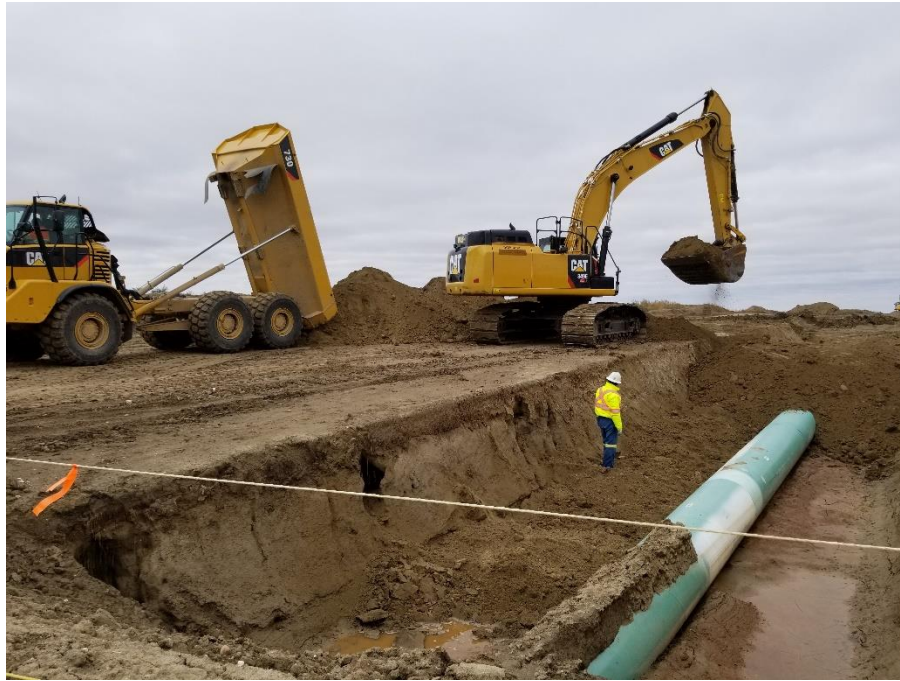
Backfilling Test point.
